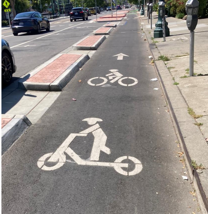
Scooter and bike icons stenciled on a Class IV separated bike lane in Oakland, CA
