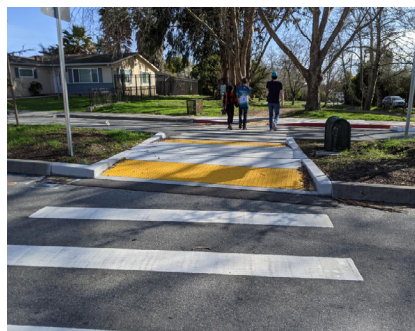
Median Refuge Island
