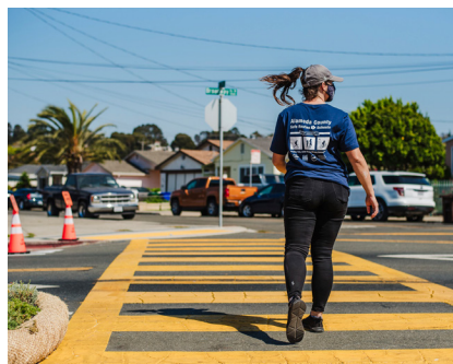
Crosswalk Visibility Enhancements
