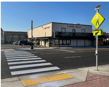
Rapid Rectangular Flashing Beacons
