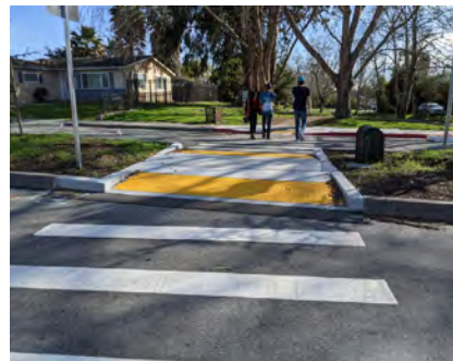
Median Refuge Island
