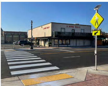
Rapid Rectangular Flashing Beacons
