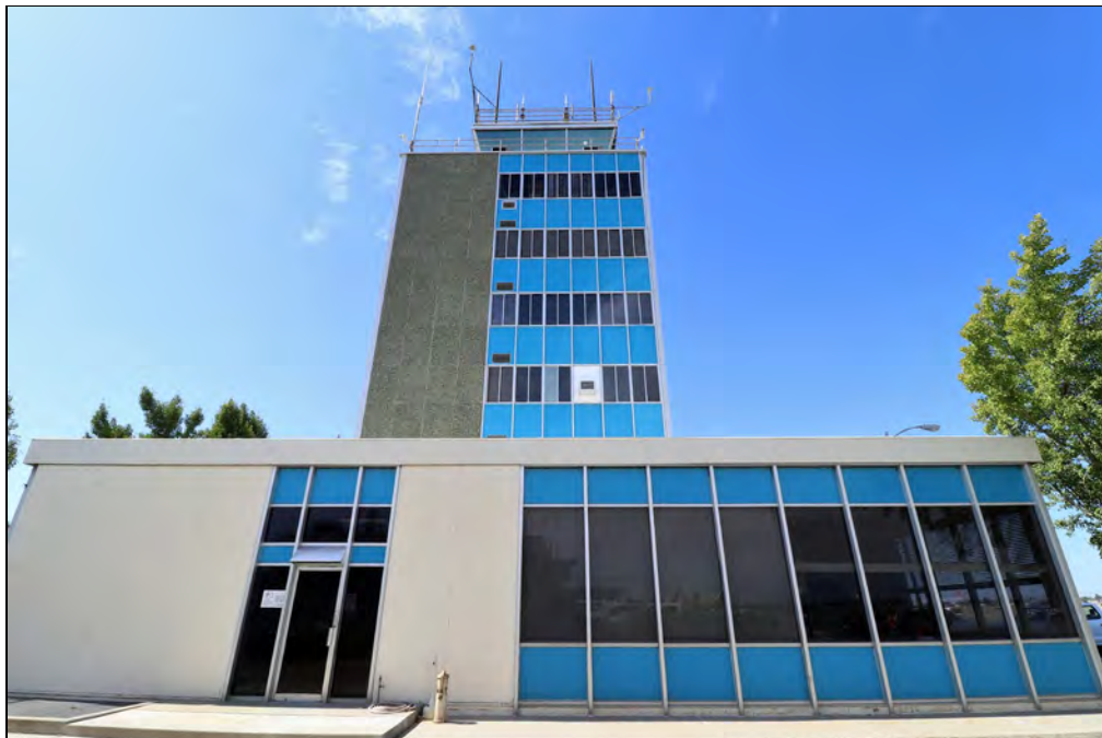
Photo 2: Southeast elevation, view northwest (9/11/23).
