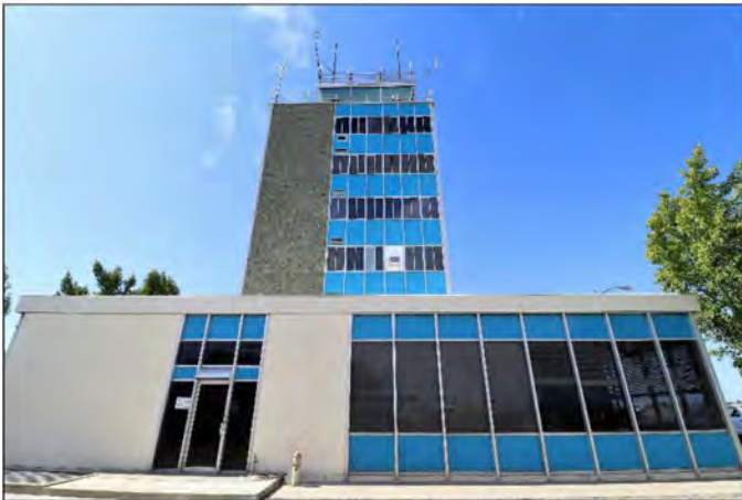
Southeast (side) elevation, view northwest (9/11/23).
