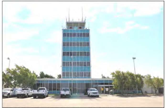
Northeast elevation, view southwest (9/11/23).
