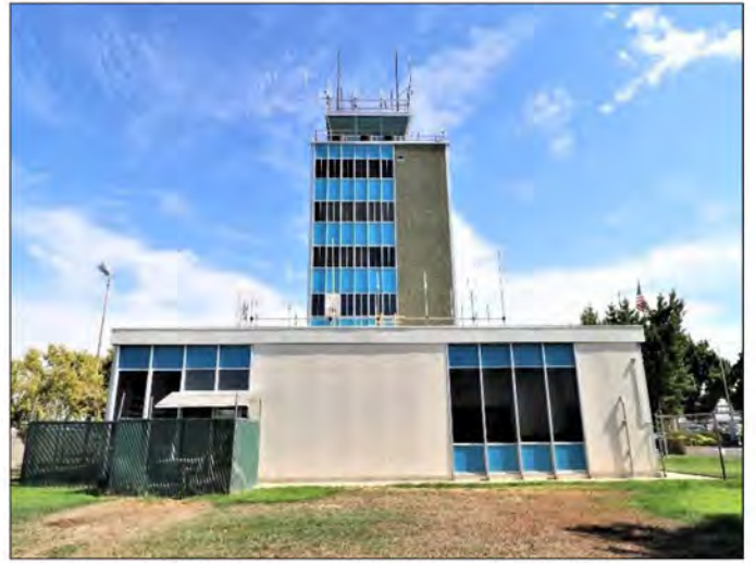
Northwest (side) elevation, view southeast (9/11/23).
