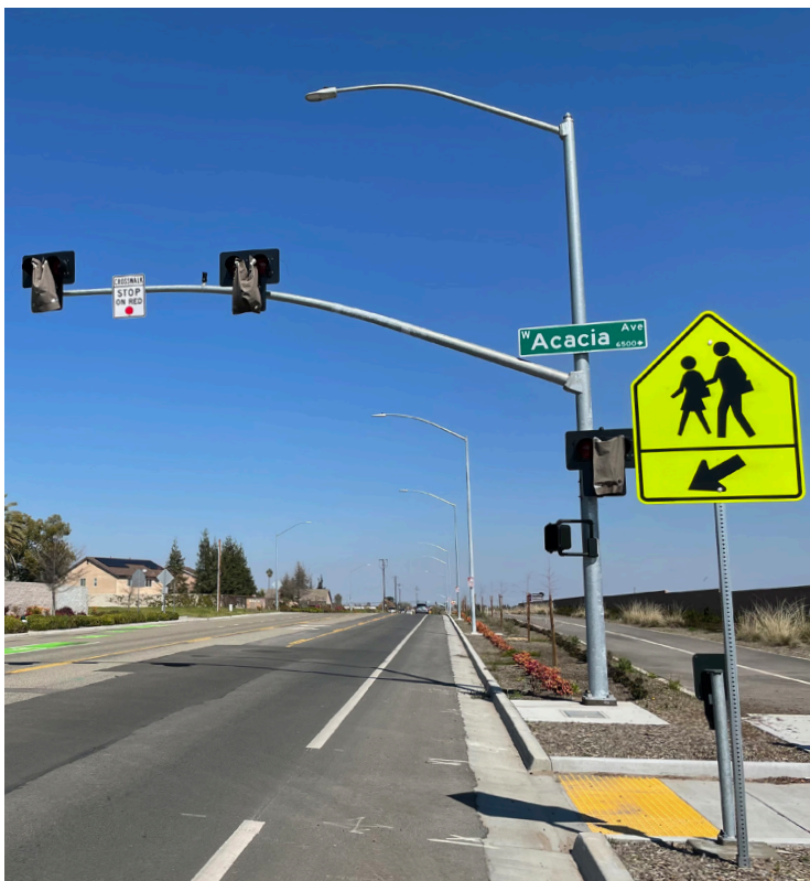
A new HAWK light being installed at the trail crossing on Bryan Avenue
