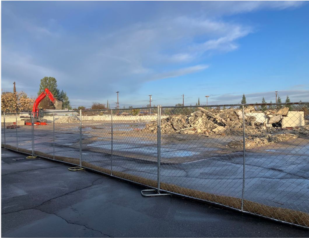
Figure 5 – Senior Center Building Demolition
