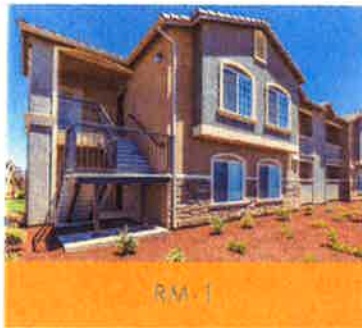
Location: Boulder Creek Builder: Spencer Enterprises
