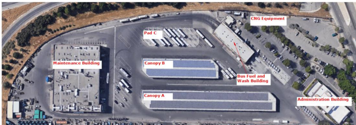
Figure 4: FAX fixed route depot (2223 G Street)
