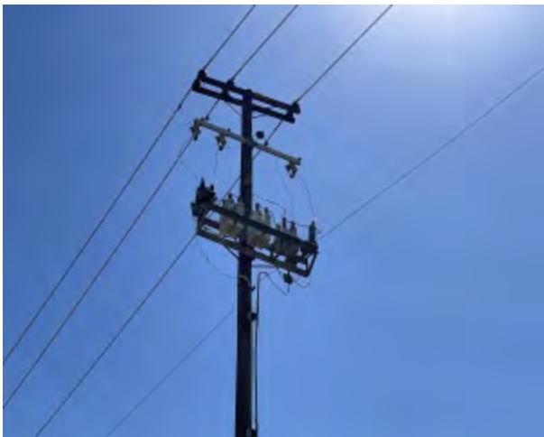
Photo 35 Comments: Triple pole mounted transformers located near south corner of building along Mono St.
