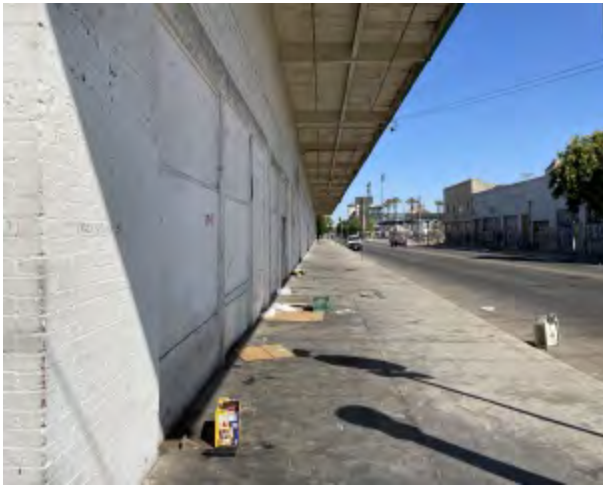
Photo 31 Comments: Exterior east corner of building looking northwest.
