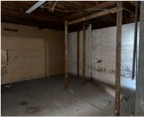
Photo 7 Comments: One of several rooms at middle of building.
