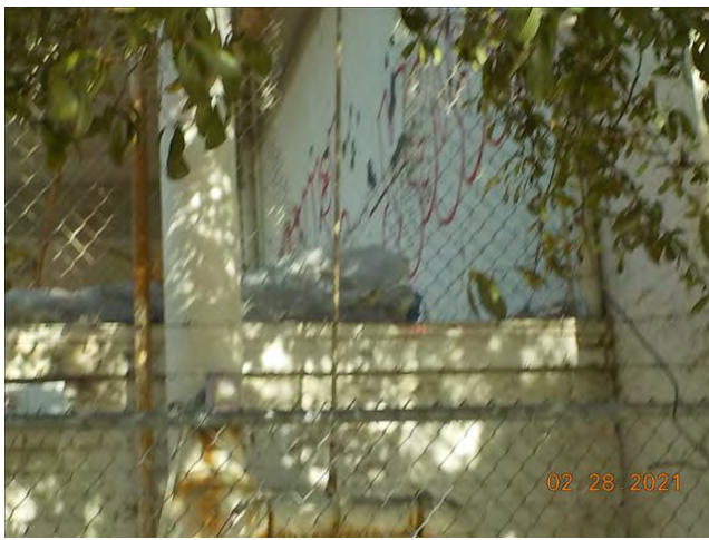
Date: 2/28/2021 9:39:01 AM ELAVATED AREA AT MONO, PHOTO TAKEN FROM MONO
