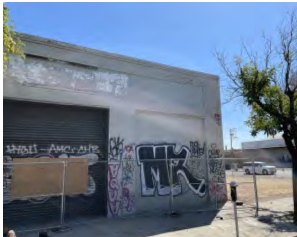
Photo 42 Comments: Strip of buildings located on northeast side of H Street. Buildings are boarded and fenced.
