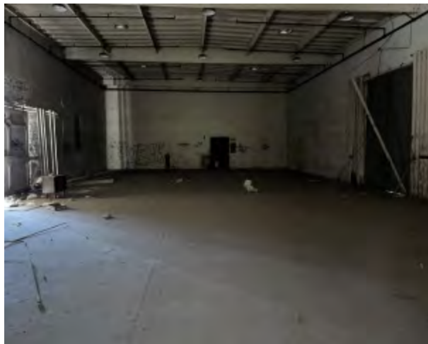
Photo 10 Comments: Third large storage area encountered moving southeast through building.
