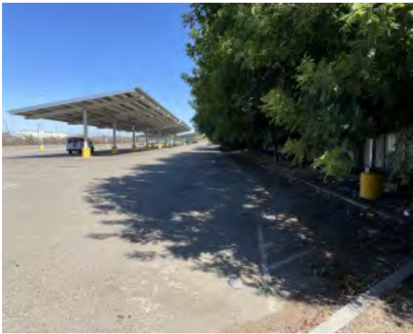
Photo 33 Comments: Near exterior south corner of building looking northwest.
