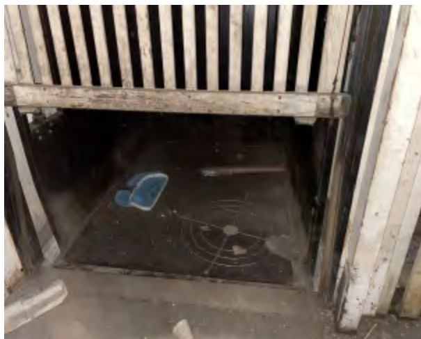
Photo 24 Comments: Basement 2 located at northwest end of building. Elevator cart.
