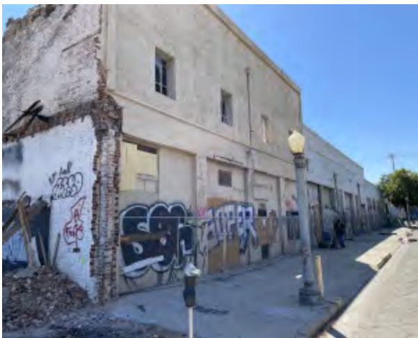
Photo 39 Comments: Strip of buildings located on northeast side of H Street. Buildings are boarded and fenced.
