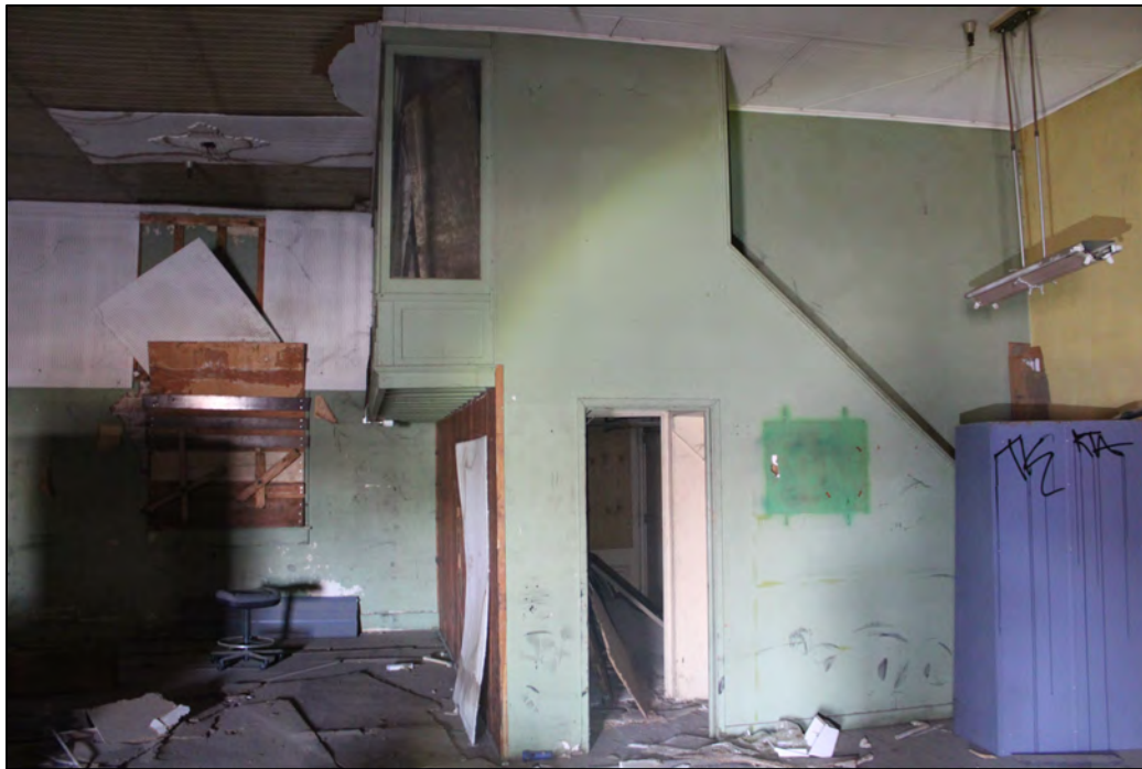
Photograph 12. Lofted office area with enclosed staircase, camera facing west, October 13, 2022.
