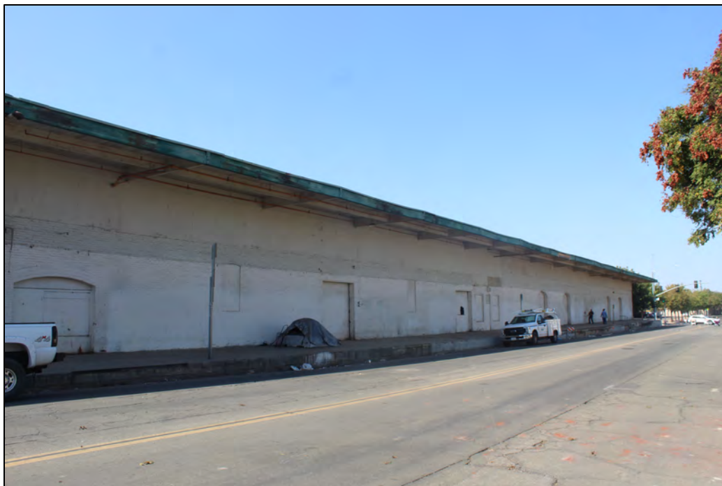
Photograph 4. Overview of 735, 739, and 741 H Street, camera facing northwest, October 13, 2022.
