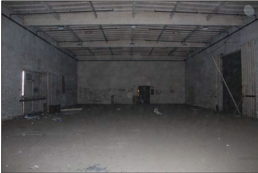
Photograph 14. Overview of warehouse interior, camera facing south, October 13, 2022.
