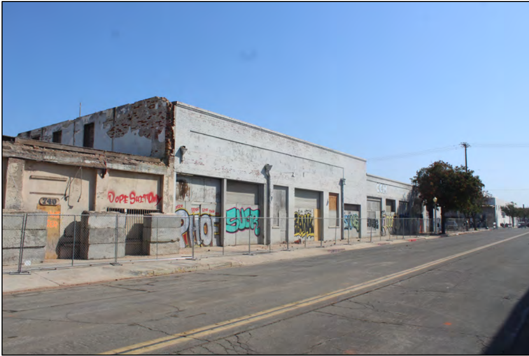
Photograph 6. Overview of 704, 710, 714, 724, and 762 H Street, camera facing southeast, October 13, 2022.
