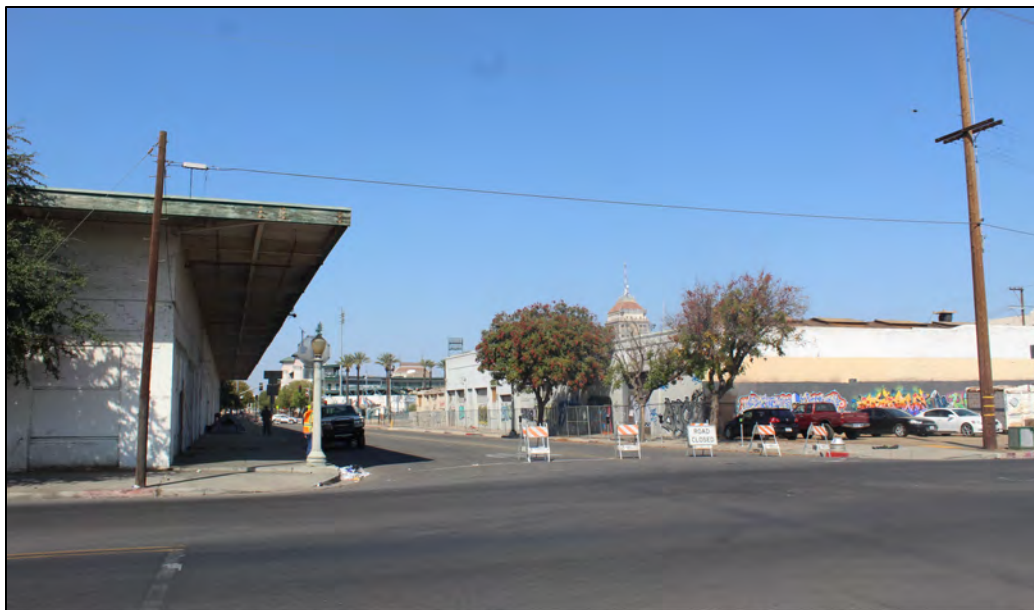
Photograph 2. Overview of intersection of H Street and Mono Street, with 735, 739, and 741 H Street on the left, camera facing north, October 13, 2022.
