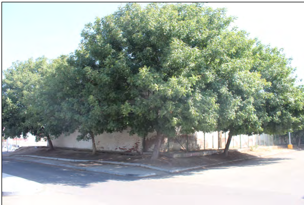
Photograph 8. Overview of north and west elevations of 735, 739, and 741 H Street, camera facing southeast, October 13, 2022.
