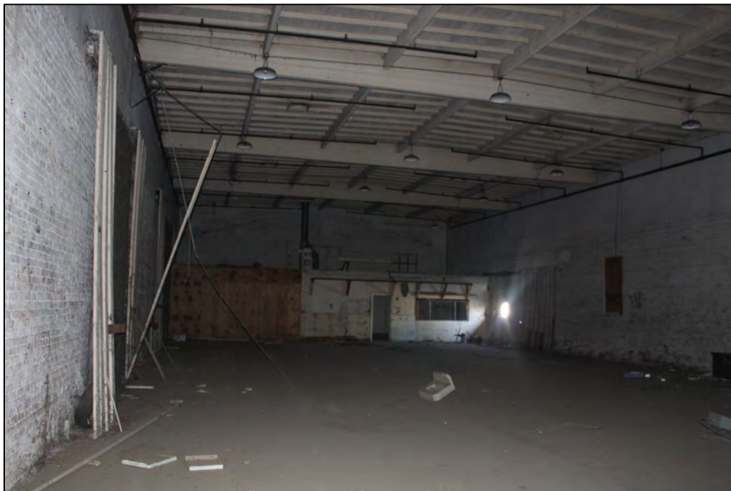
Photograph 15. Overview of warehouse interior, camera facing north, October 13, 2022.
