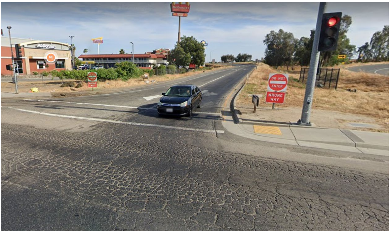
FIGURE 14: JENSEN AVENUE FACING SOUTH AT SR 99 NORTHBOUND OFF-RAMP
