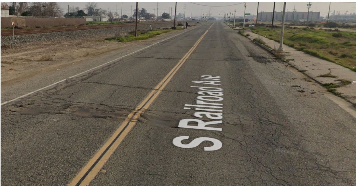
FIGURE 16: RAILROAD AVENUE FACING SOUTH
