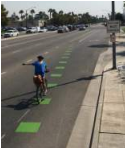
Figure 15: Green Colored Pavement on Palm Avenue
