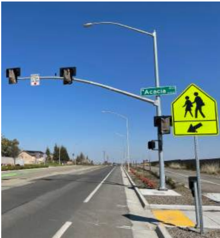
A new HAWK light being installed being installed at the trail crossing on Bryan Avenue
