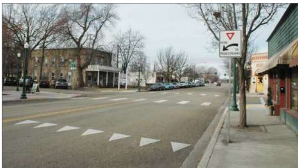
Advanced "shark teeth" yield line before a pedestrian crossing.
