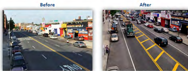
Example of a Road Diet on Southern Blvd, Bronx, NY Source: NYCDOT
