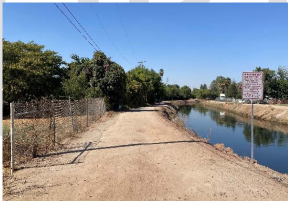
Figure 6. Typical canal bank conditions
