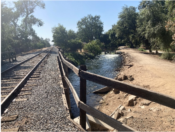
Figure 10. Railroad crossing of canal
