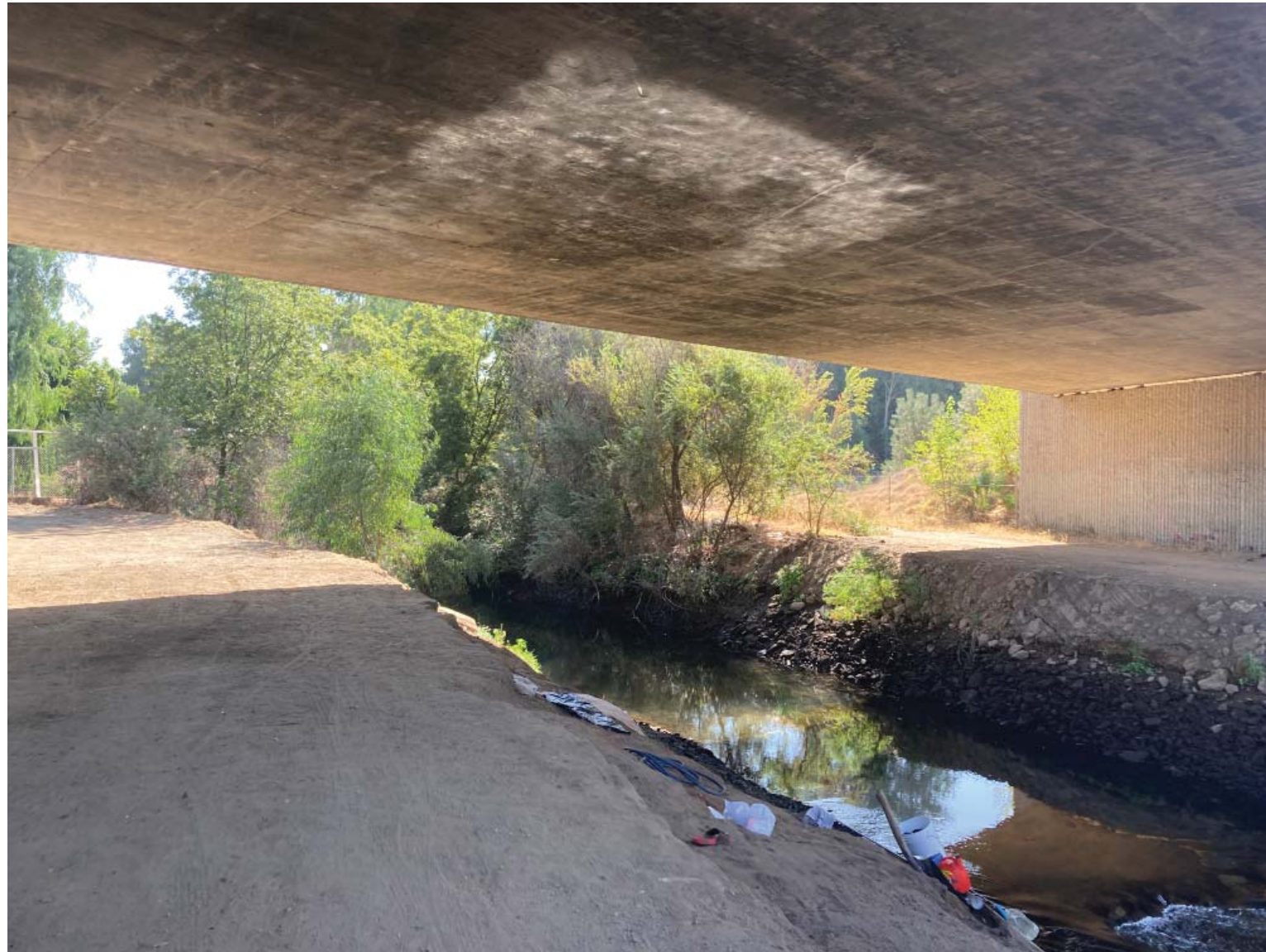
Looking east from north bank under Hwy 180 overpass
