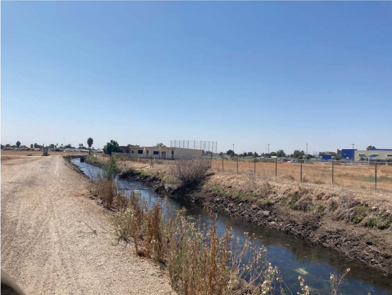
Looking south from Church, with school building visible on right
