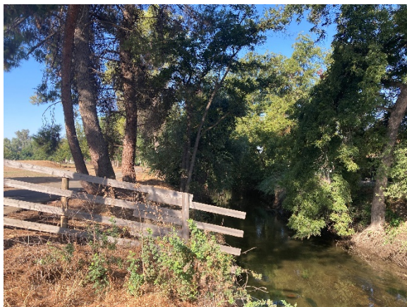
Figure 8. Example of private property/encroachment
