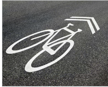
Figure I.4: A 'sharrow' symbol used to indicate a shared travel lane (image: Flickr user - drdul)
