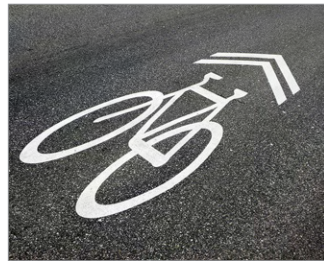
Figure 5.12: A ‘sharrow’ symbol used to indicate a shared travel lane (image: Flickr user - drdul)
