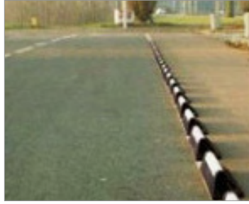
Figure 5.15: Vertical delineators provide a buffer to the adjacent traffic lane (image: Northern Green Technologies, LLC)
