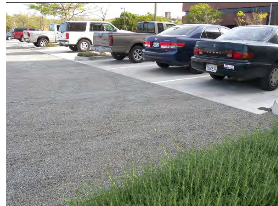
The use of pervious paving, which is lighter in color than asphalt, in parking lots helps significantly reduce stormwater runoff during the rainy season and surface temperatures during the hot summer months.
