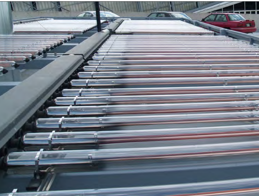
Solar evacuated tube collectors generate green power.
