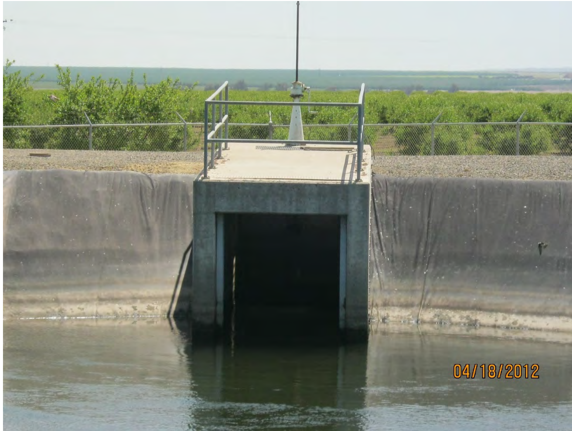
Figure Q.6: Lateral 1R-4.0-1.0C Sunk Intake Structure
