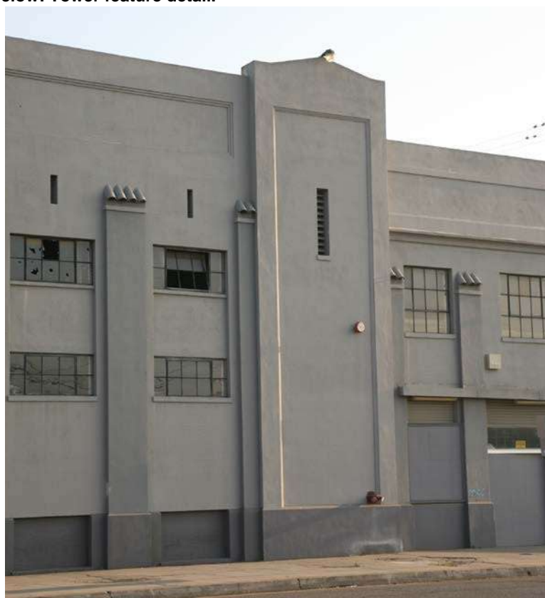
Above: Detail of pilasters, tile caps and industrial sash windows. Below: Tower feature detail.
