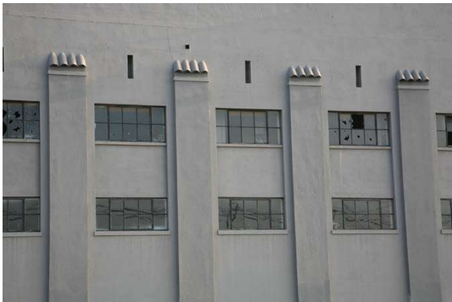
Above: Detail of pilasters, tile caps and industrial sash windows. Below: Tower feature detail.
