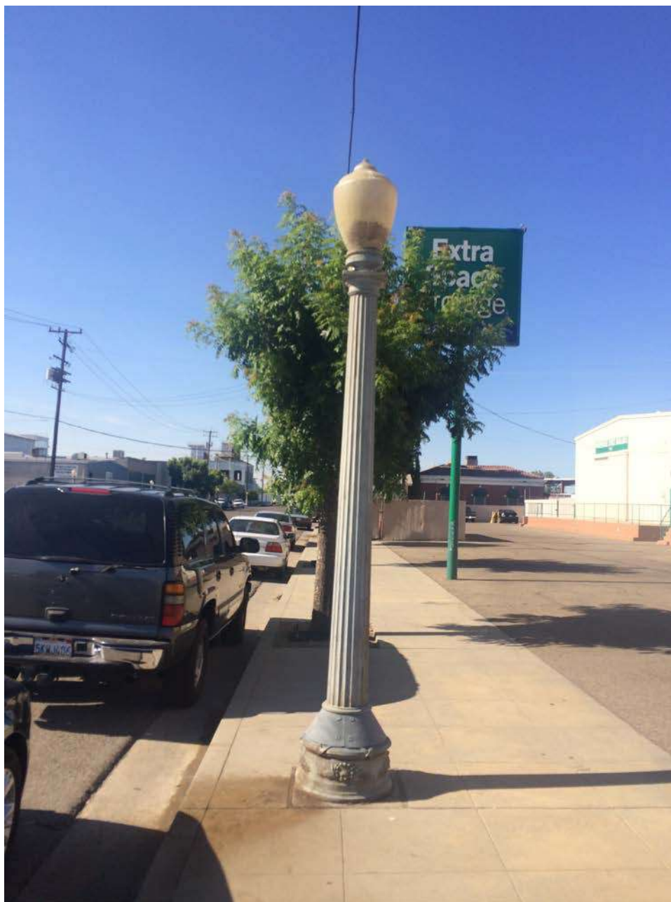
P5b. Description of Photo: Squat standard on S. Cherry Ave. looking South. Bases are Union Metal Lamp Standard Design No. 649.
