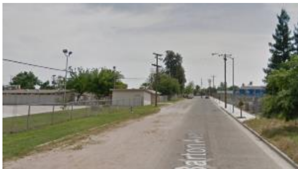
Example of missing and incomplete sidewalk segments along Barton Avenue
