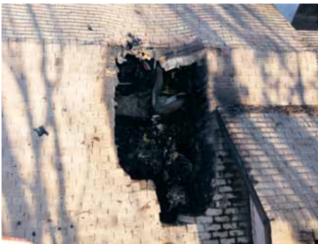
Location of roof failure
