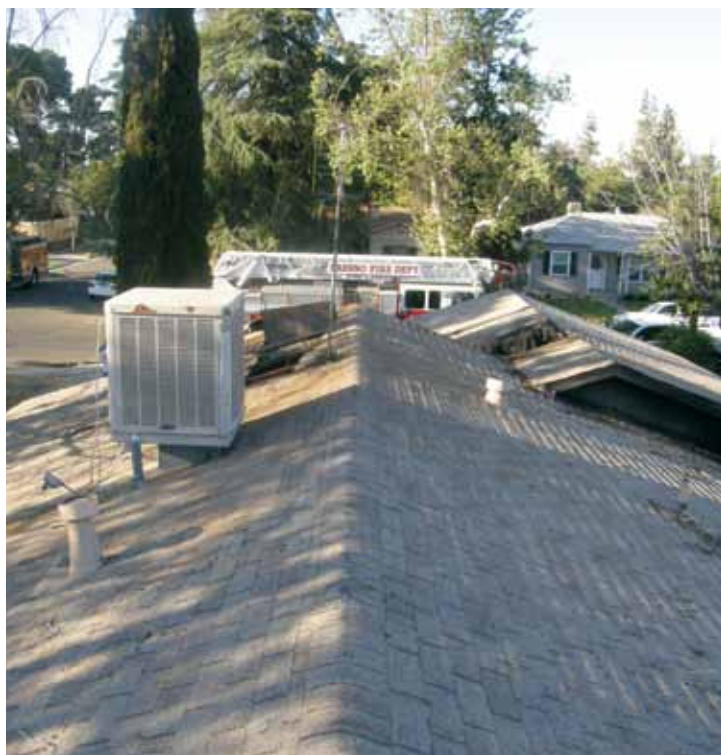
View of roof from the south
