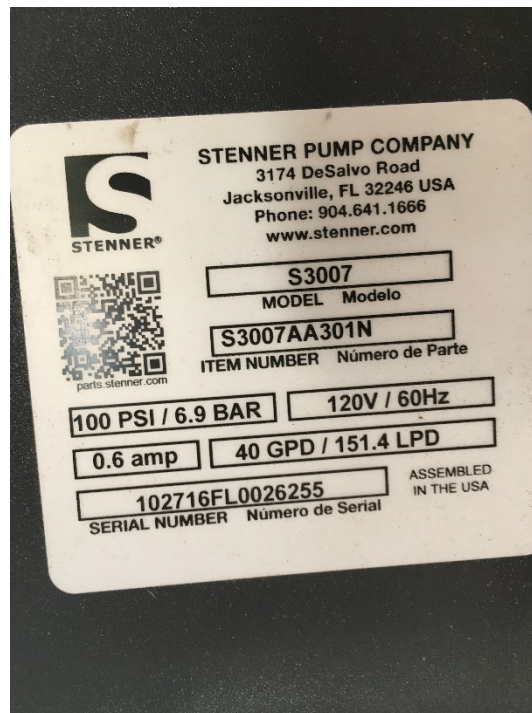
Figure 4.35: Chlorine Dosing Pump Nameplate
