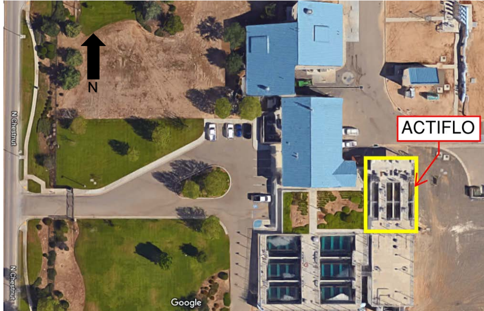
Figure 5.13: Site View with Highlighted Actiflo Units.
