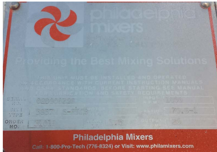
Figure 5.20: Flocculation Mixer Nameplate
