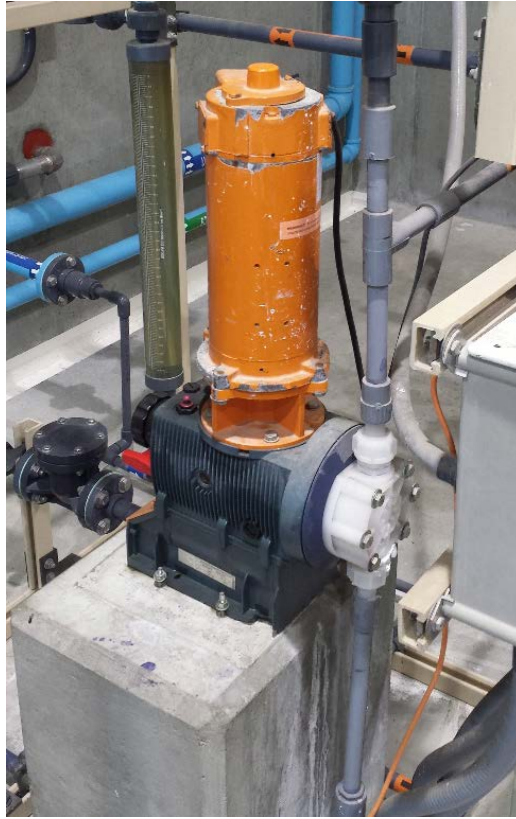
Figure 5.71: Polyphosphate Feed Pump
