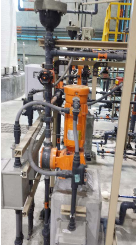
Figure 5.62: Alum/Ferric Feed Pump System
