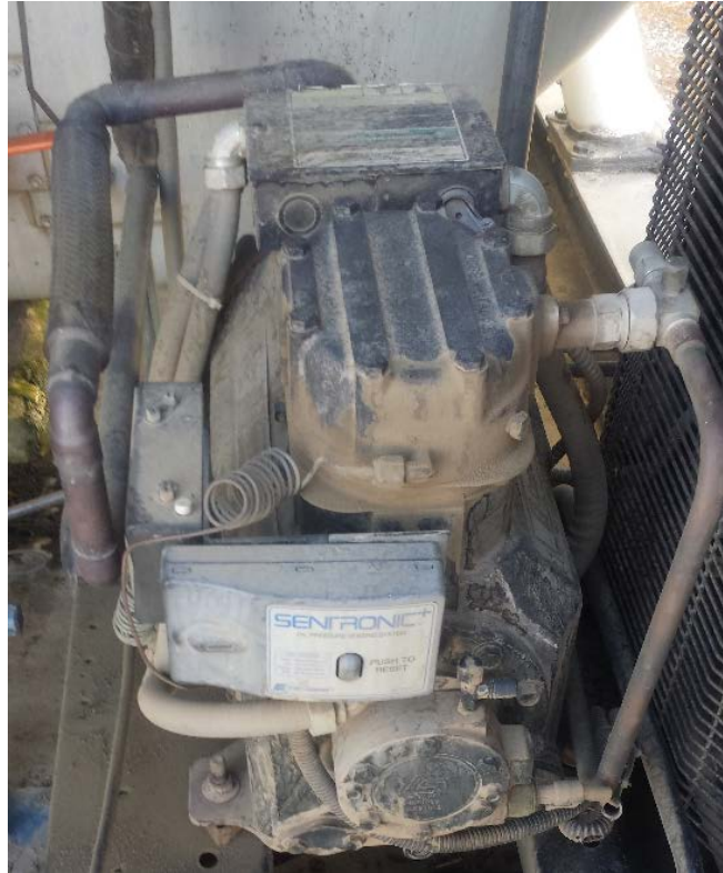
Figure 5.74: Vaporizer Compressor
