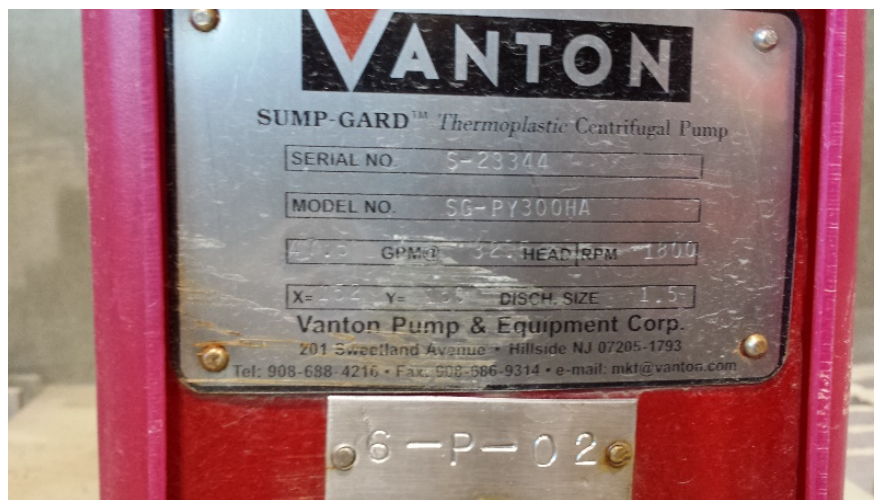
Figure 5.76: Chemical Sump Pump 6-P-02 Nameplate
