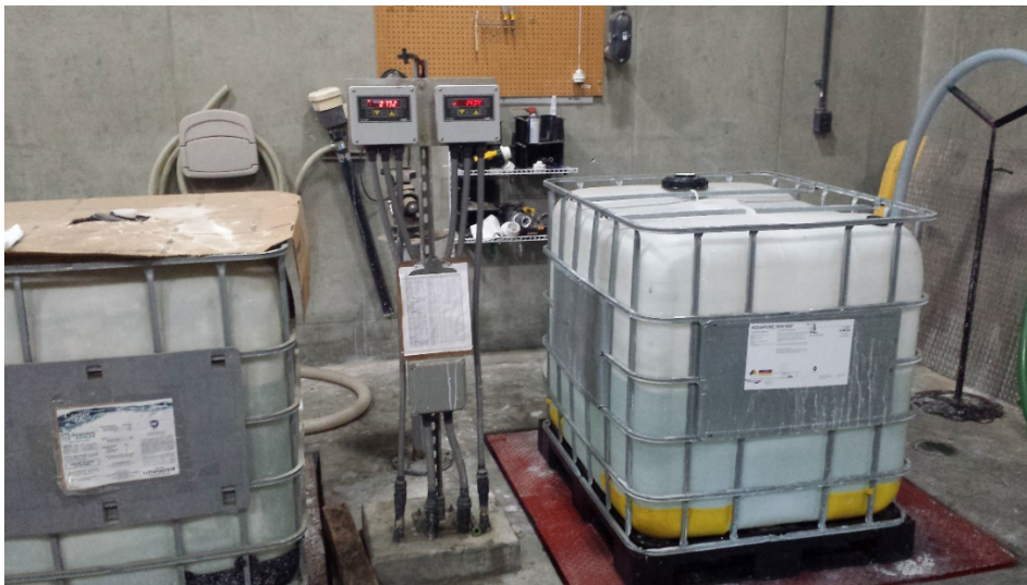
Figure 5.69: Weigh Scales for Polyphosphate
