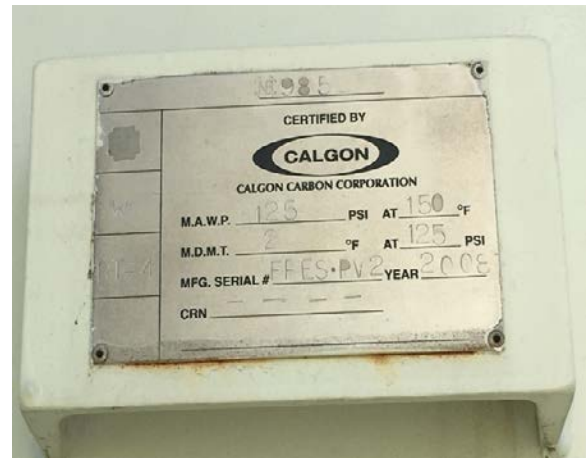
Figure 4.9: GAC Vessel 2 Name-plate
