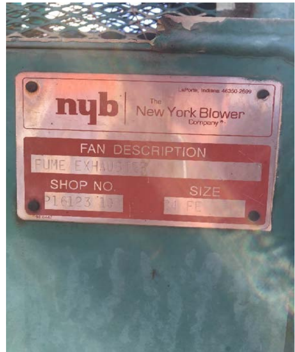
Figure 4.55: Air Blower Nameplate
