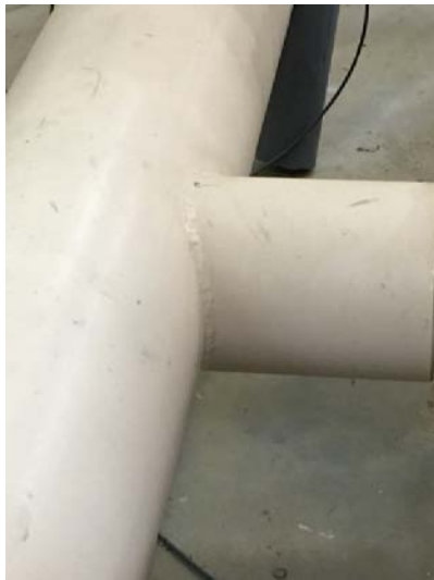
Figure 4.24: Welded Tee Connection Between Wells 184 & 225
