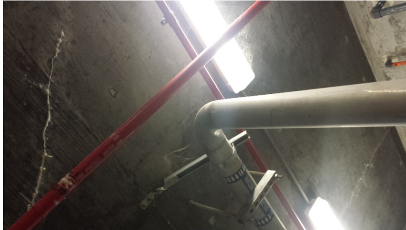
Figure 5.28: Ceiling of Solids Pump Room
