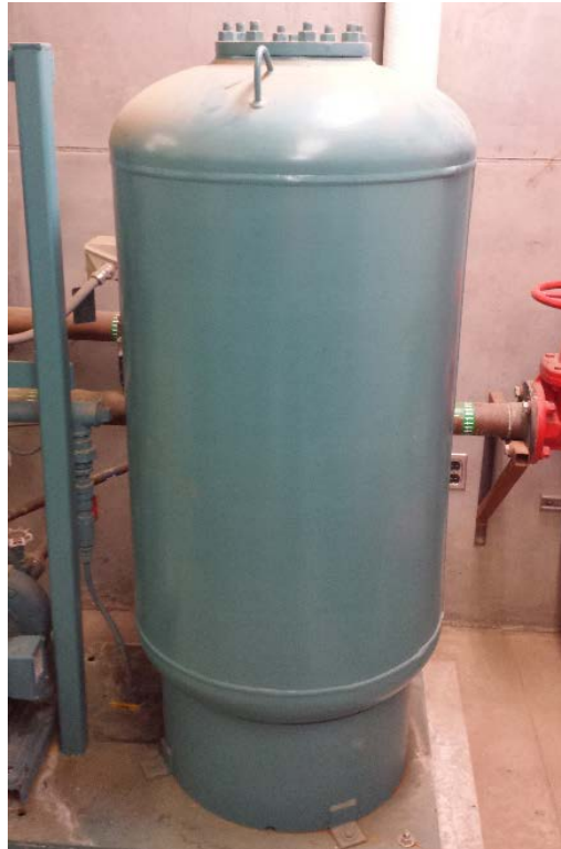
Figure 5.80: Pressure Vessel
