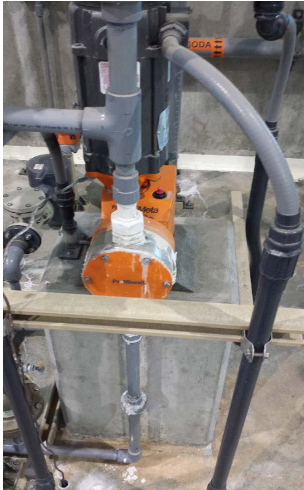
Figure 5.66: Feed pump caustic system
