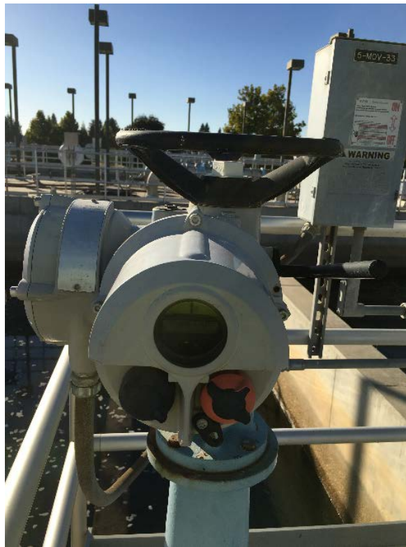
Figure 5.46: Drain Valve Actuator
