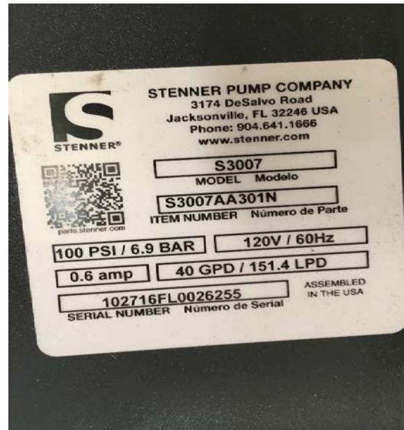
Figure 4.37: Chlorine & Orthopolyphosphate Dosing Pump Nameplate
