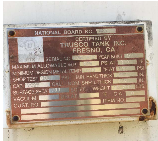
Figure 4.63: GAC Vessel 2 Nameplate
