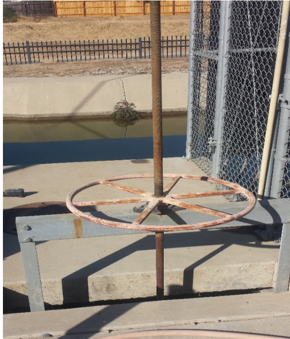
Figure 5.4: Inlet Gate Top View
