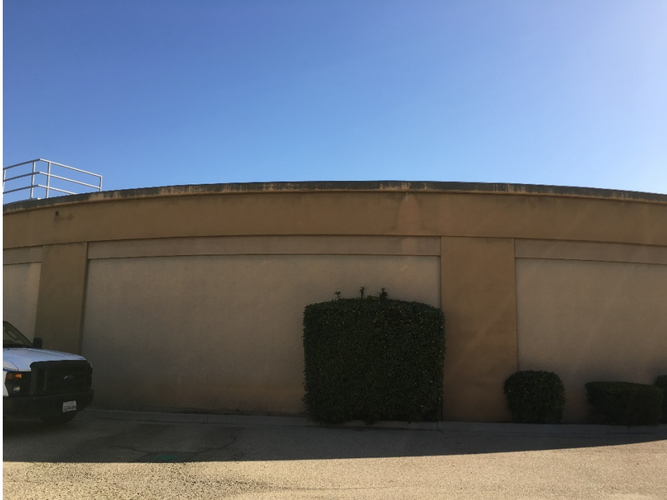
Figure 4.27: 2-MG Storage Tank at Wellhead Site 225
