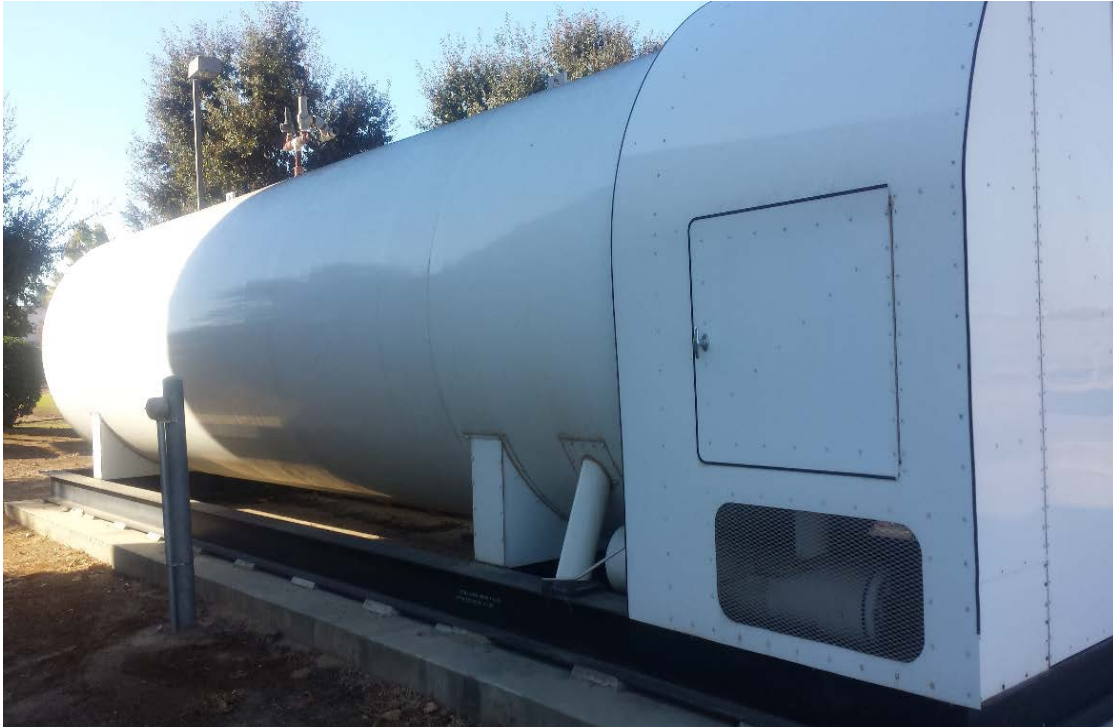
Figure 5.72: Carbon Dioxide Storage Tank
