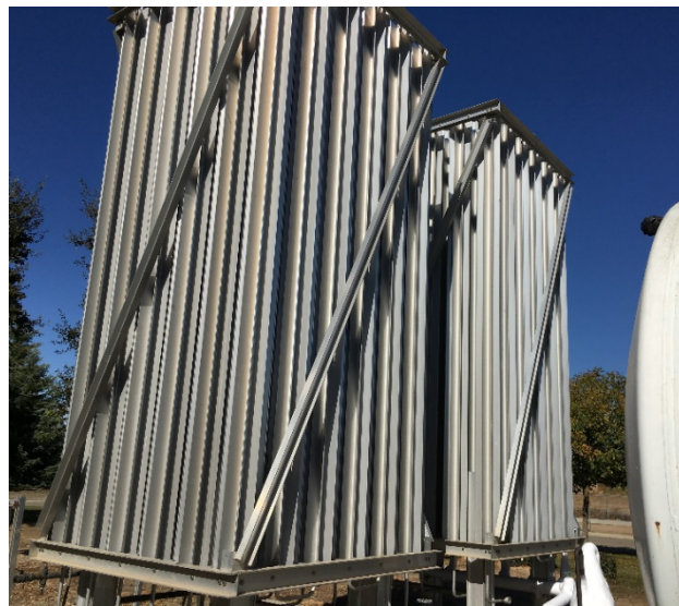
Figure 5.35: Vaporizer Units
