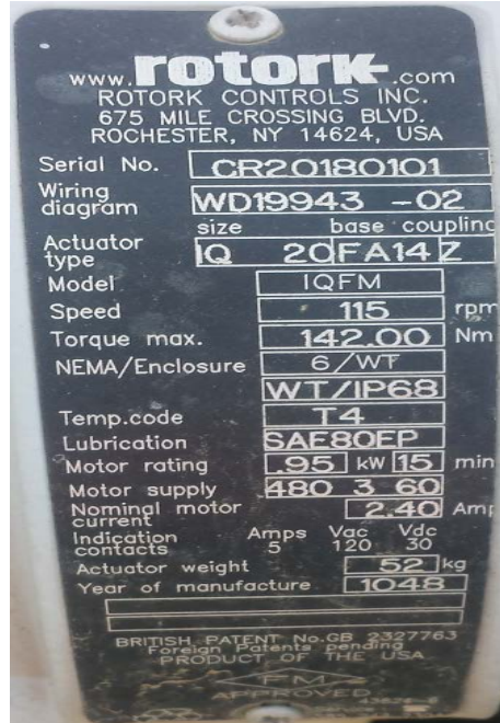
Figure 5.5: Diversion Gate Electric Actuator Nameplate
