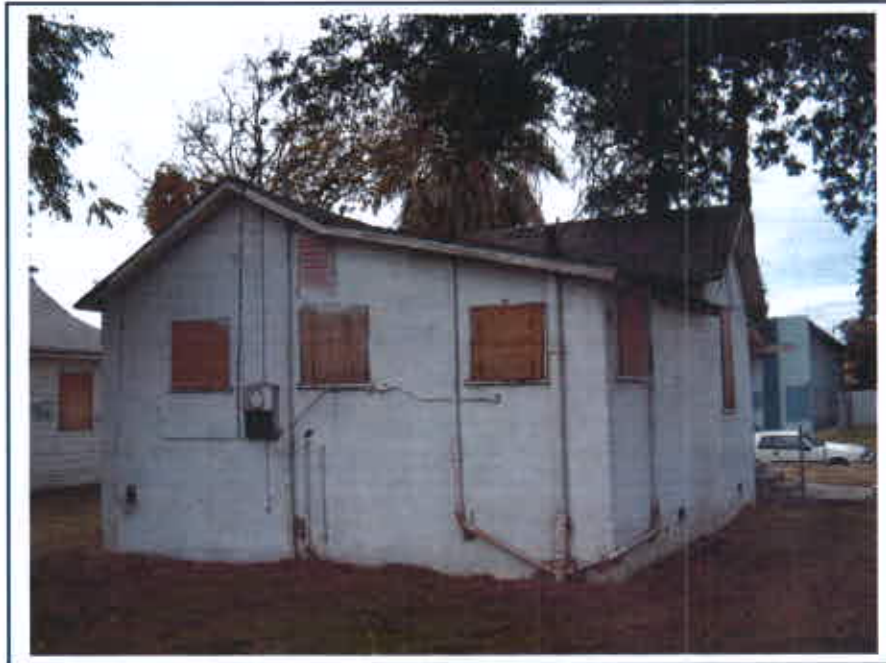
East (Rear) Elevation of 172 N. Echo Avenue
